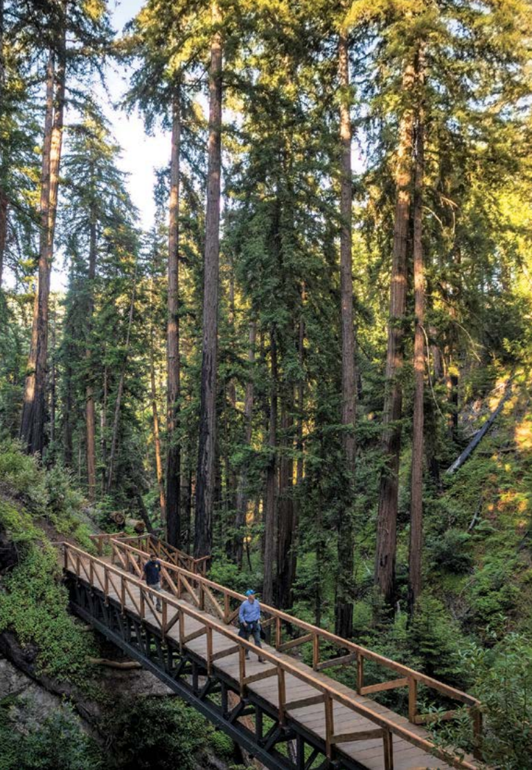
The renovated Pfeiffer Falls Trail in Pfeiffer Big Sur State Park winds through the redwoods and features a 70-foot pedestrian bridge.
